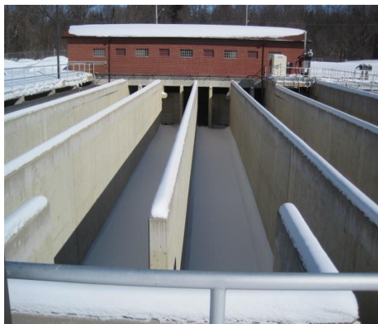
Chlorine Contact Chamber
