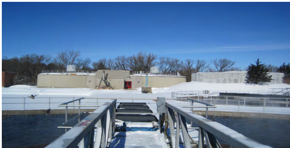
2 Stage Anaerobic Digestion (Primary on the left and Secondary on the right, boiler room in the middle)
