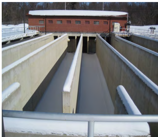
Chlorine Contact Chamber
